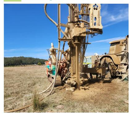
Clay + high water flow = mud Mud + river gravel = clogged line Mud + gravel + hard dolerite = X#\$!
