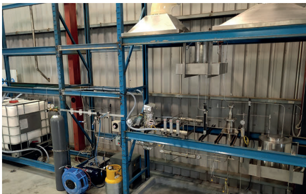
Image: The first stage of the Alcore pilot plant facility
