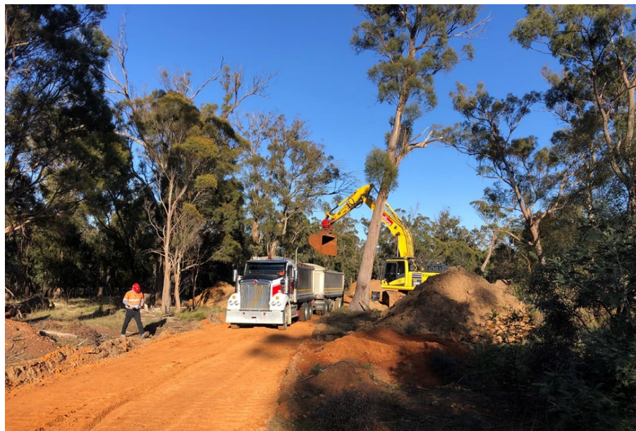
Fingal Rail bauxite operations November 2021
