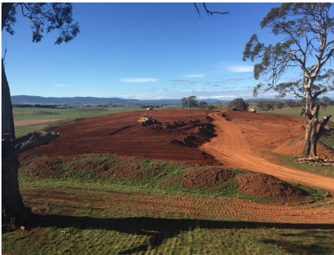
Mine and screening sites being rehabilitated October 2016
