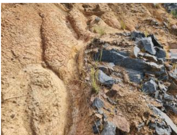
Figure 7: Example of the mixed drilling environment of hard rock boulders, wet clays and bedrock
