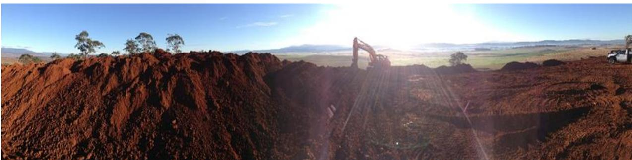
**Figure 5: Each run-of-mine bauxite stockpile is from a single bench from a specified pit for product management**
