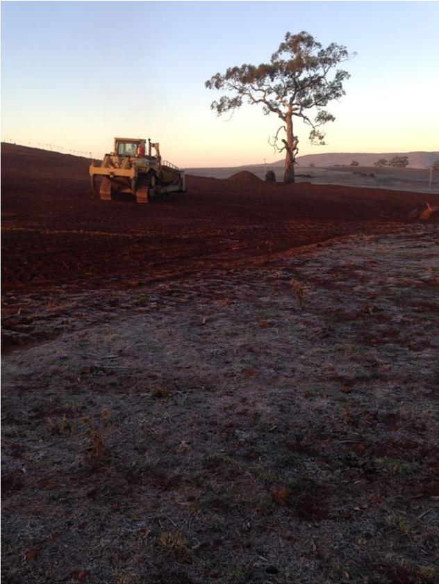
**Figure 3: Stripping thin topsoil early on frosty mornings eliminates dust. Operator skills & methods have improved due to experience & common sense.**
